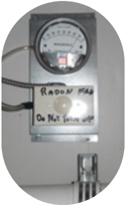
The second gauge that may be found on radon mitigation systems is an electric Magnehelic Differential Pressure Gauge (MDPG) and will have a switch indicating “Radon Fan, DO NOT TURN OFF”.
