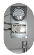
The second gauge that may be found on radon mitigation systems is an electric Magnehelic Differential Pressure Gauge (MDPG) and will have a switch indicating "Radon Fan, DO NOT TURN OFF".
